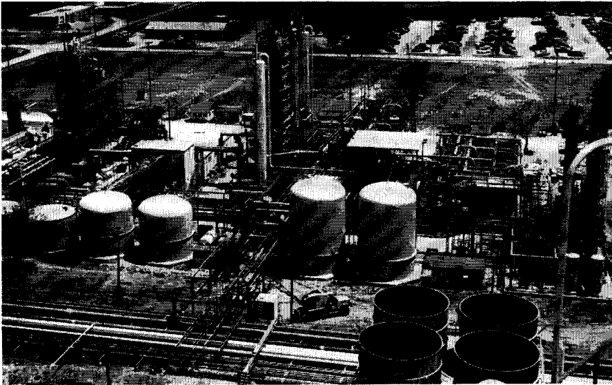
Cyanamid's new Offier plant near New Orleans, now producing sulfuric acid, ammonium sulfate, and oxygen, will soon go stream to make acetylene, anhydrous ammonia, hydrocyanic acid, and acrylonitrile.
